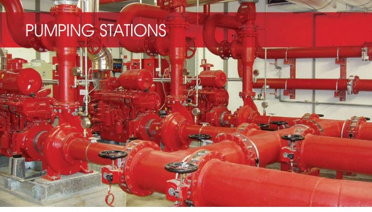
The pumping station is at the heart of every stationary extinguishing system. This is where the necessary pressure is generated for the extinguishing water and downstream extinguishing areas and units.
