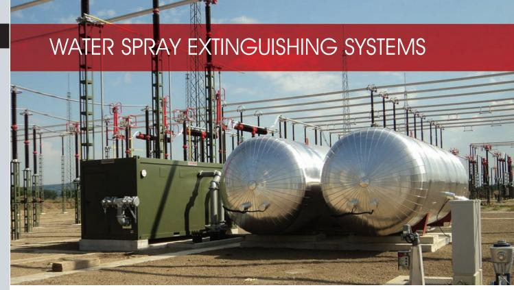
Water spray extinguishing systems protect objects and rooms which are susceptible to fire outbreaks. Whilst sprinkler systems selectively spread extinguishing water over the fire when necessary, water spray or water deluge systems can be used to extensively spray, cool and therefore protect larger technical objects. Furthermore, the flue-gas cleaning effect offers excellent personal protection in the event of a fire.
